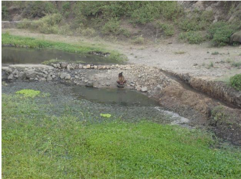
Figure 1. Checkdam type water abstraction on small streams (Majete)
