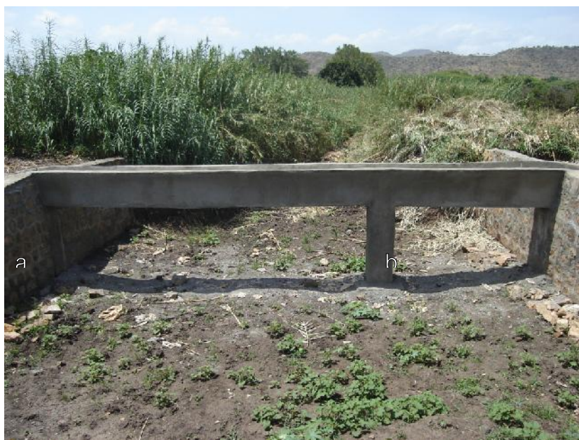
Figure 3. Irrigation canal crossing hill (a-Bakelo) and water way(b-Shewarobit)
